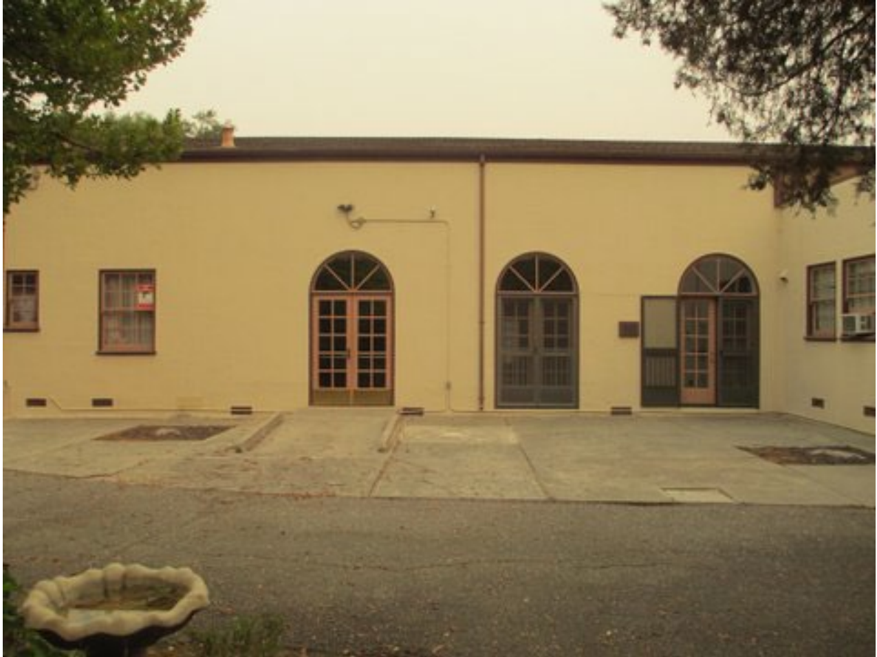
Photo No. 5 of 11: South Elevation looking North
