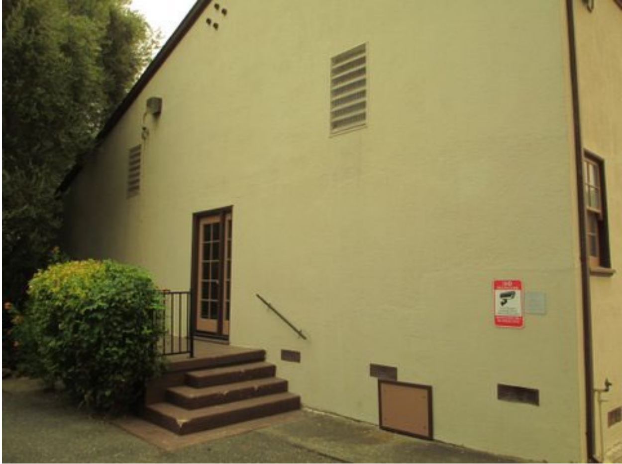
Photo No. 6 of 11: West Elevation looking Northeast
