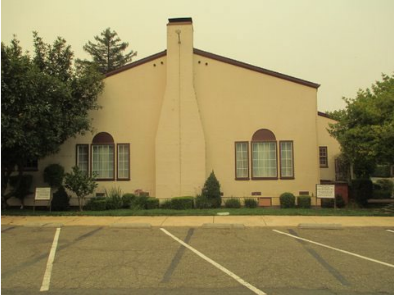
Photo No. 4 Of 11: East Elevation looking West
