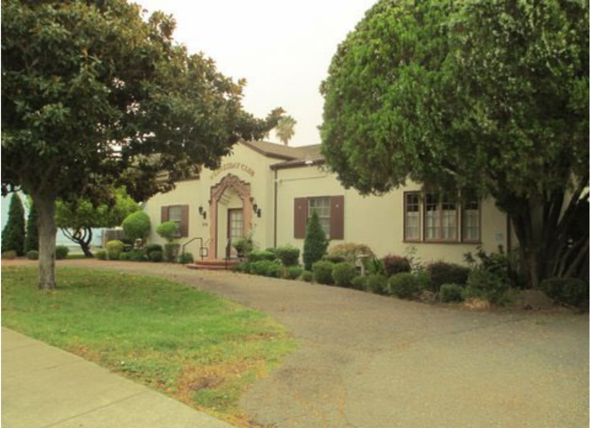
Photo No. 3 of 11: North Elevation looking Southeast
